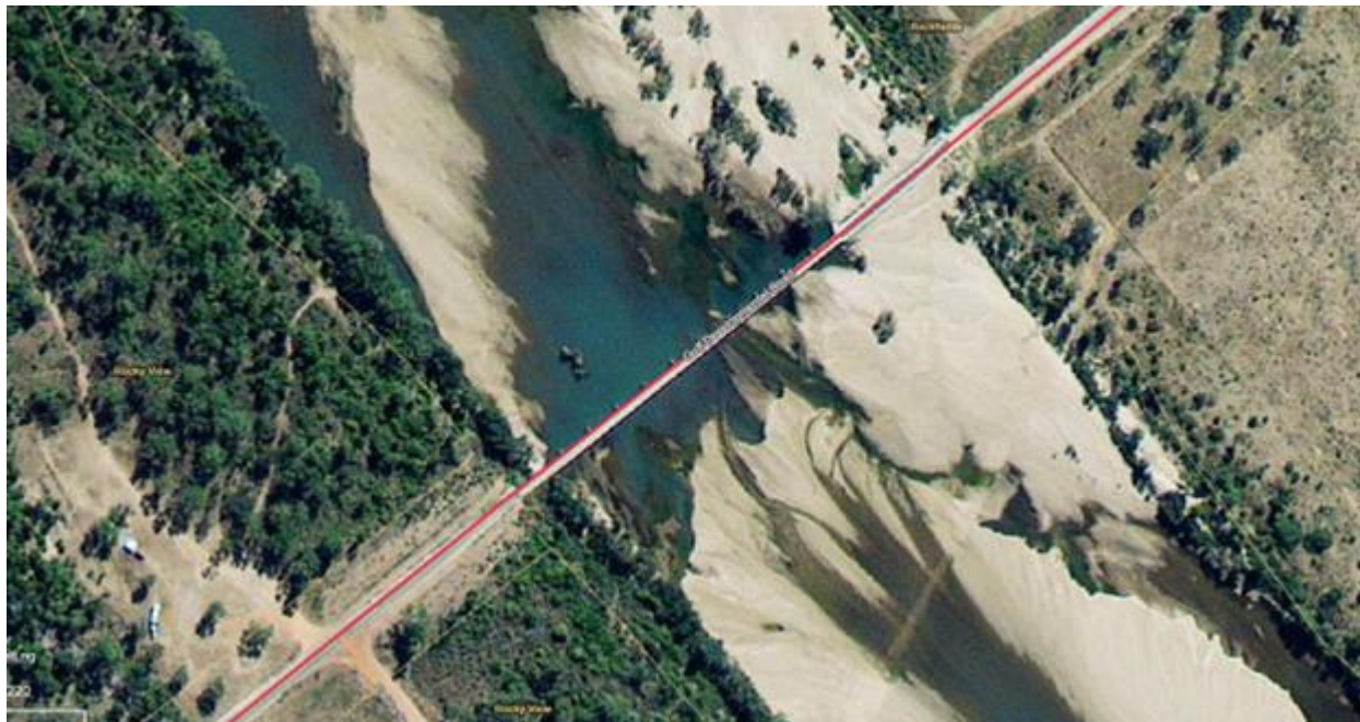
Figure B-7: Gilbert River bridge crossing
